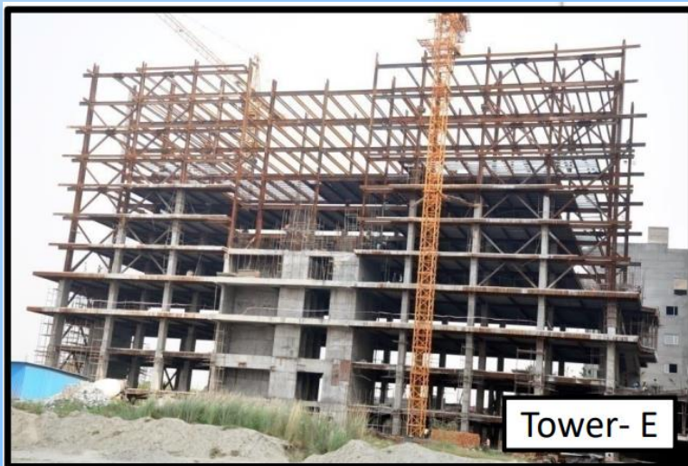
Steel structure starts to go up while concrete encasing is done on below floors
