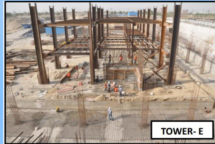
Two storey structure steel erected
